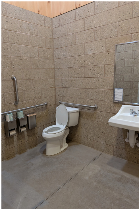
Figure 7 Toilet Room at the Pavilion
