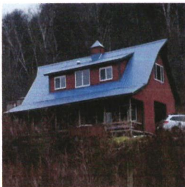
Post & Timber Barn w/ Steel Siding/Roof – interior unfinished.
