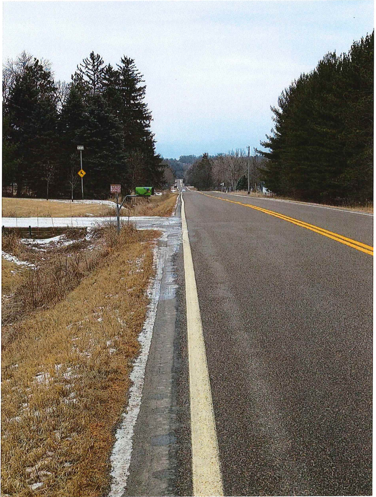
Image is facing north from proposed new access driveway location
