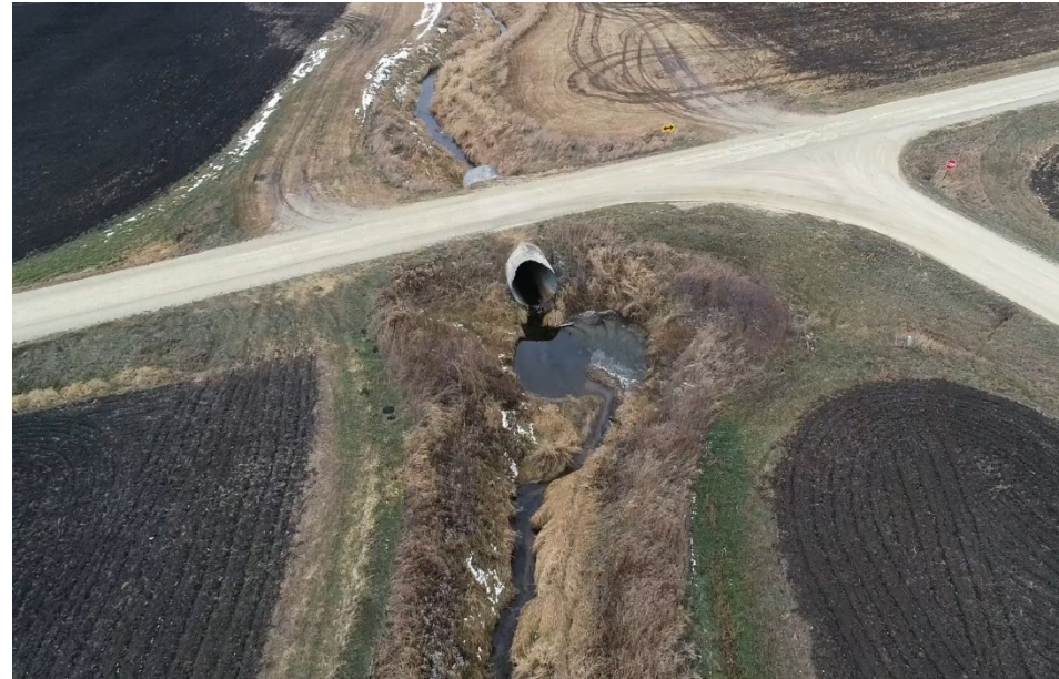
Culverts Above Channel
