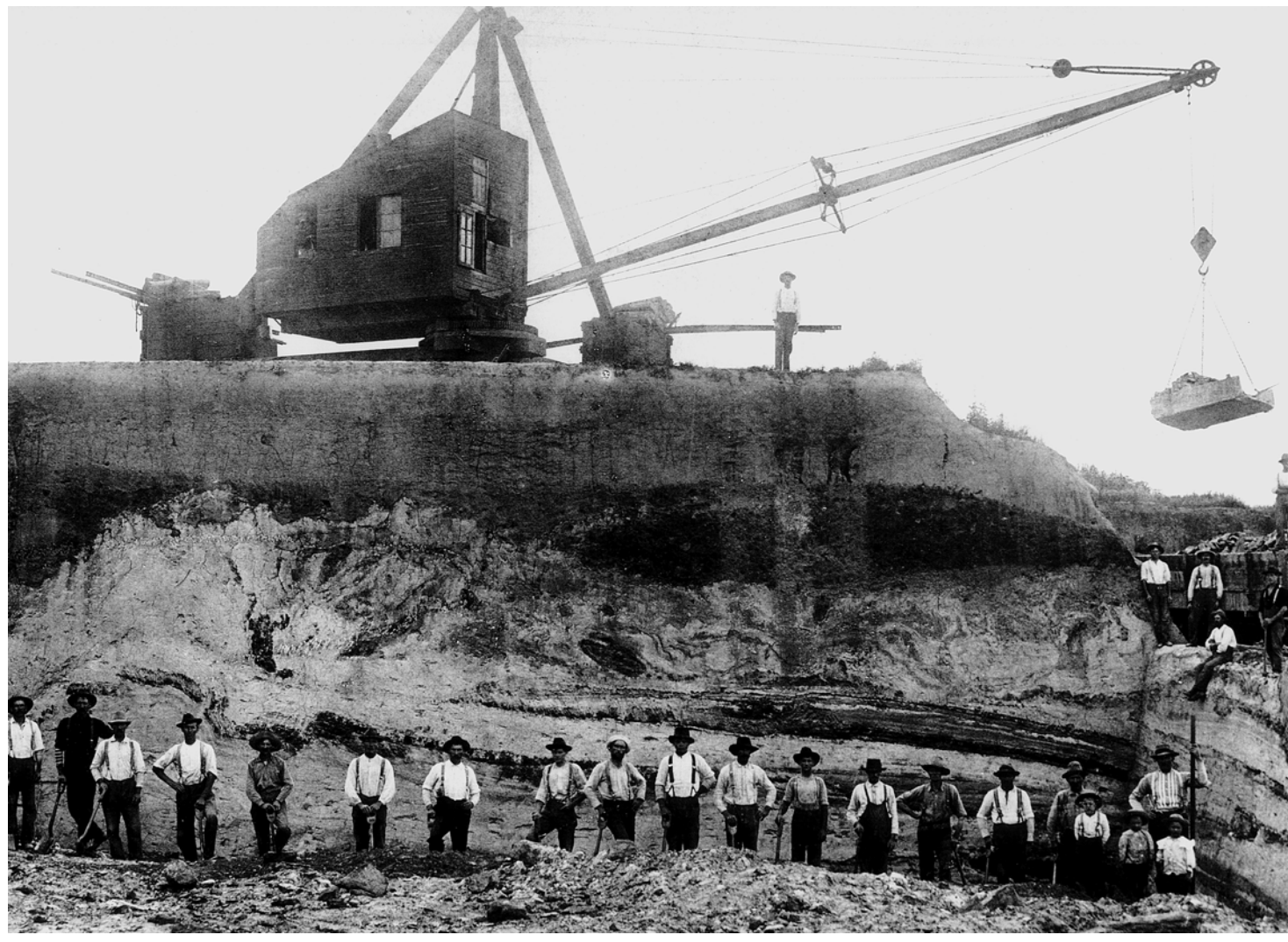
Figure 1. A Goodhue County clay pit at the turn of the century. Miners used shovels to dig the clay and place it in the buckets, which were lifted out of the pit by the derrick. From the historical photographic collection of Phil Revoir, Red Wing, Minnesota (published with permission).
