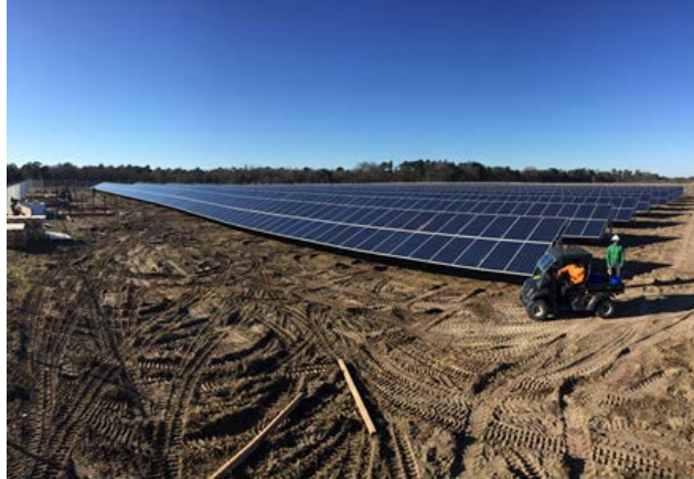
EXAMPLE OF A SOLAR PROJECT IN CONSTRUCTION
