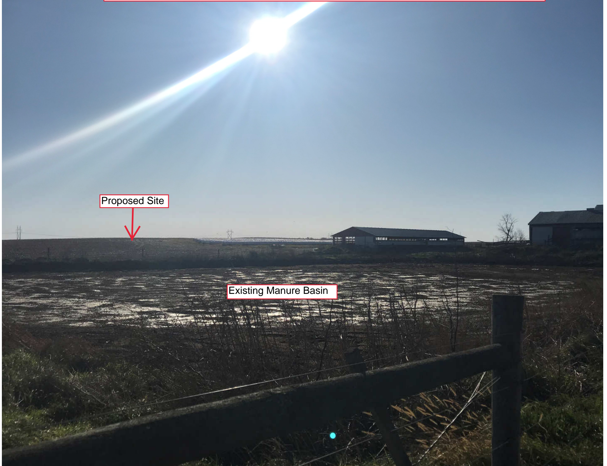
Photo #5 - Existing manure basin and proposed new site looking from northwest to southeast.
