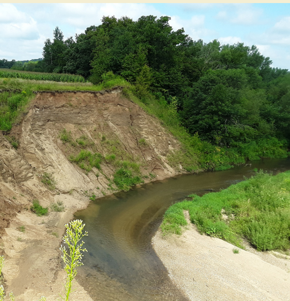
Streambank erosion on Mazeppa Creek near the confluence with the North Fork of the Zumbro River
