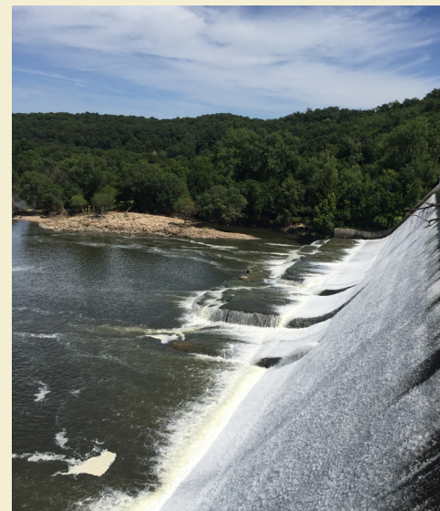
Water flows over the spillway of Lake Zumbro Dam.
