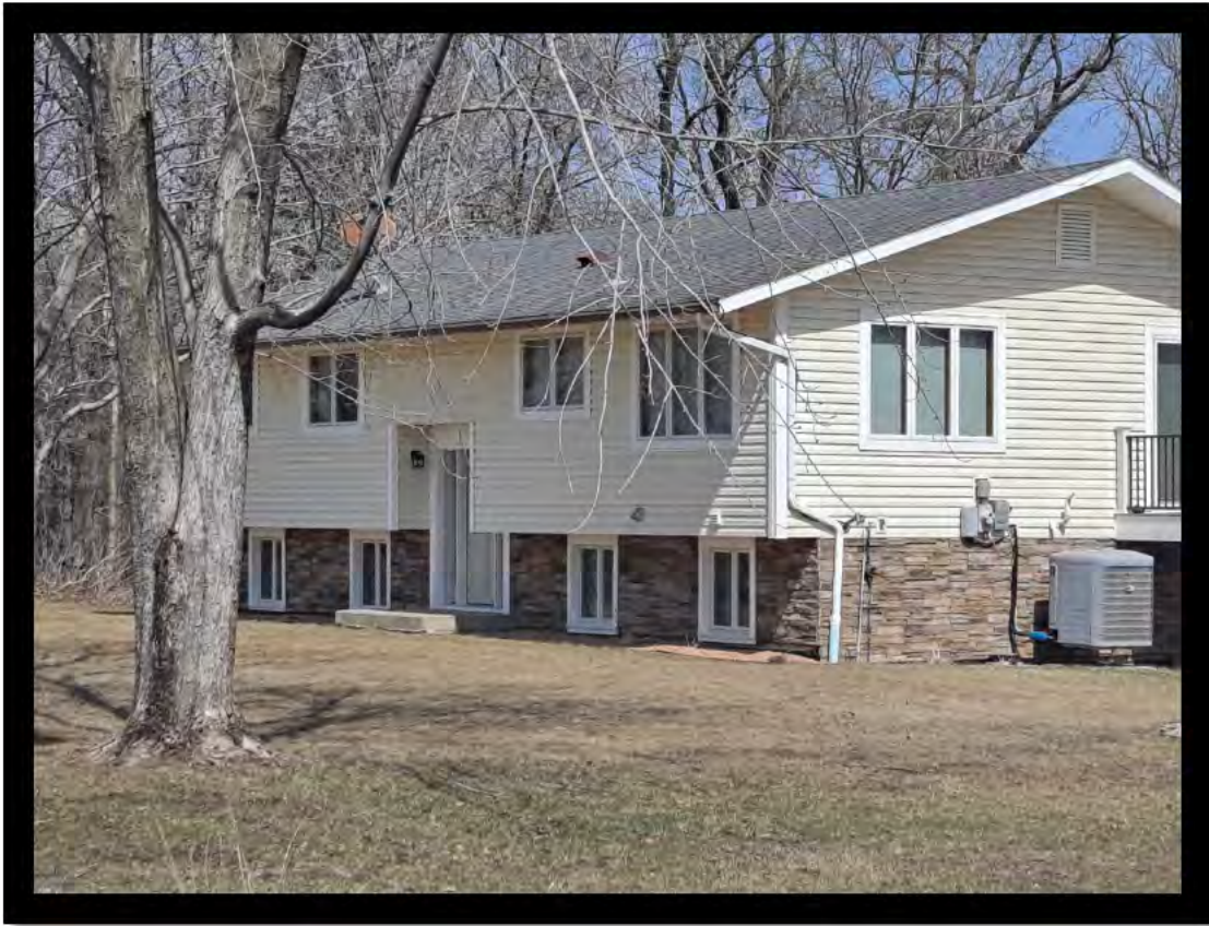
Utilities enter the home on the south side.
