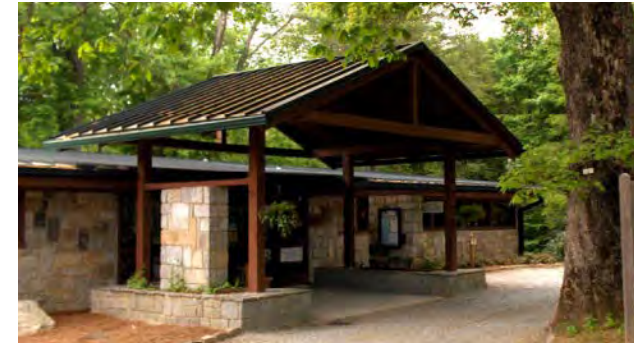
The Learning Lab building
