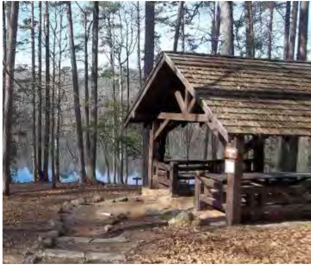
Rustic Picnic Shelter & Overlook
