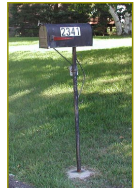
2-inch diameter metal pipe
